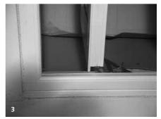
4) By closing the sash the hinges return to the fire egress position automatically.
