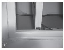
4) By closing the sash the hinges return to the fire egress position automatically.
