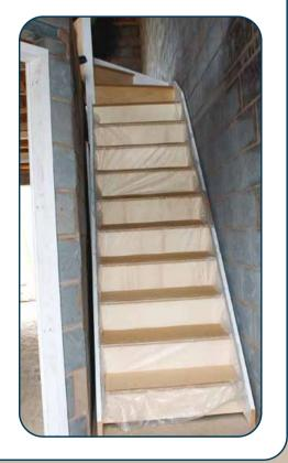
Make sure glue blocks are glued on all loose risers. Screw and glue winder treads to newel posts making sure at all times the newel is square to the last tread and loose wall string is square to main string.
